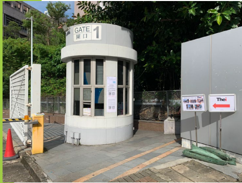
Access Gate 1 at Sai Shan Road 由細山路1號閘口進入
